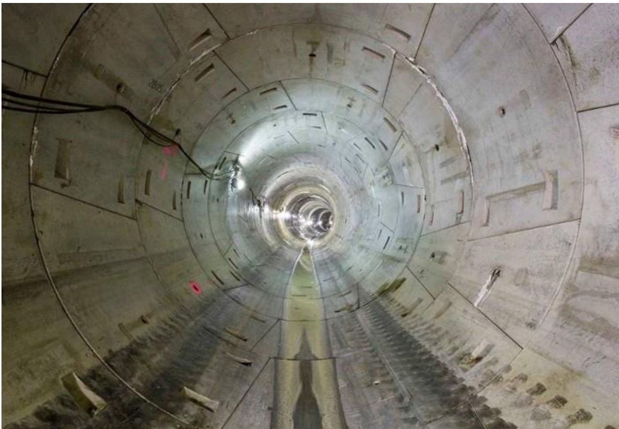
Figure 4. Example Pre-cast Concrete Segmental Lining
