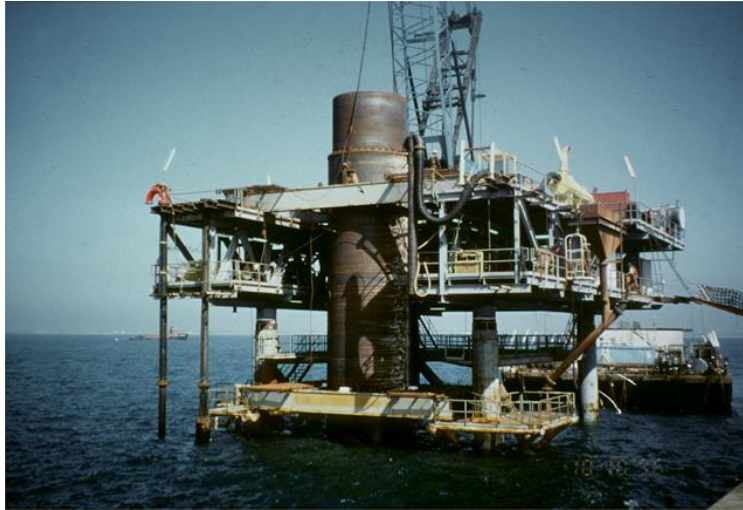
Figure 7. Example of a Vertical Conveyance Shaft Being Lowered Toward a Tunnel at Sea
