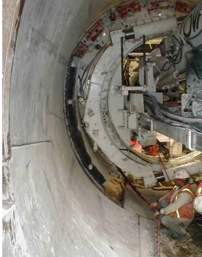
Figure 5. EPB TBM Erecting a Pre-cast Concrete Segment
