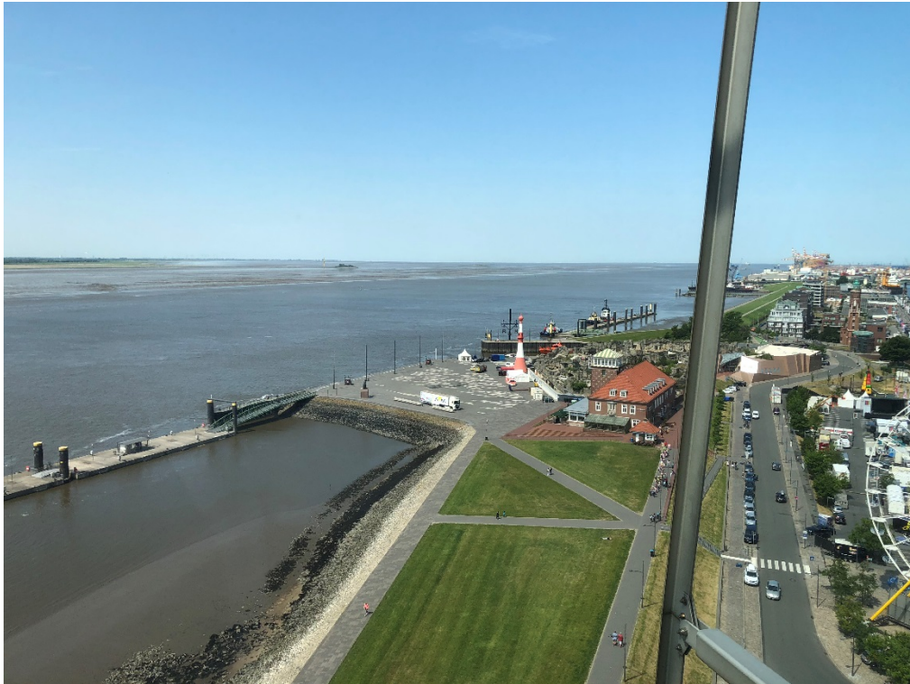
Port of Bremerhaven – View of ship channel commingled with residential area.
