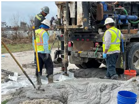
Photo 9 Advancement of boring at DMMU-3-2B / DMMU-4-2B, facing southwest.
