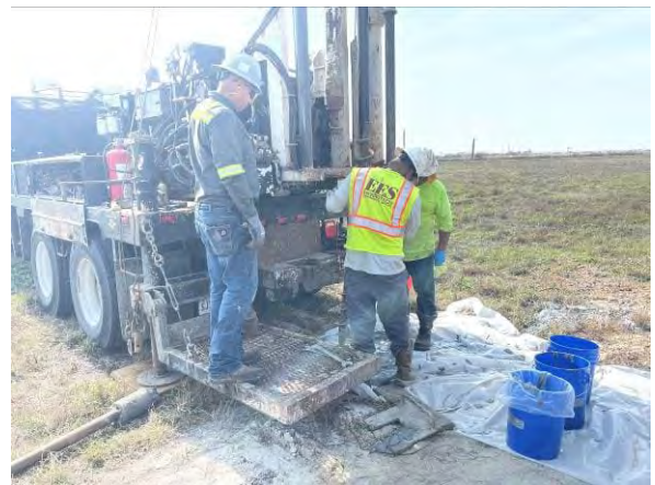
Photo 6 Advancement of boring at DMMU-5-3B / DMMU-6-3B, facing southeast.
