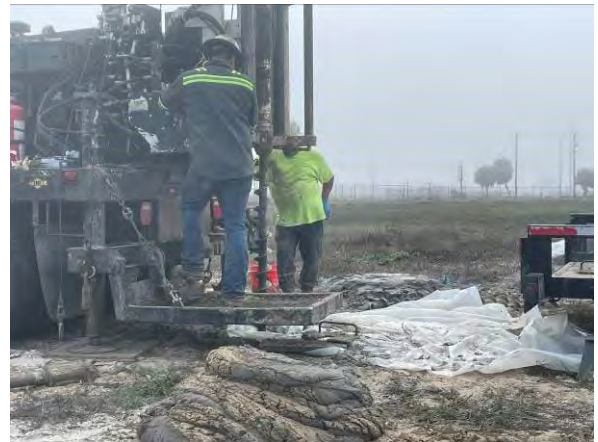
Photo 4 Advancement of boring at DMMU-1-1C / DMMU-2-1C, facing southeast.
