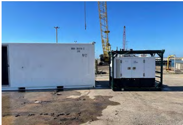
Photo 15 View of refrigerated unit at Martin Energy facility used to store samples at or below 4°C following collection.
