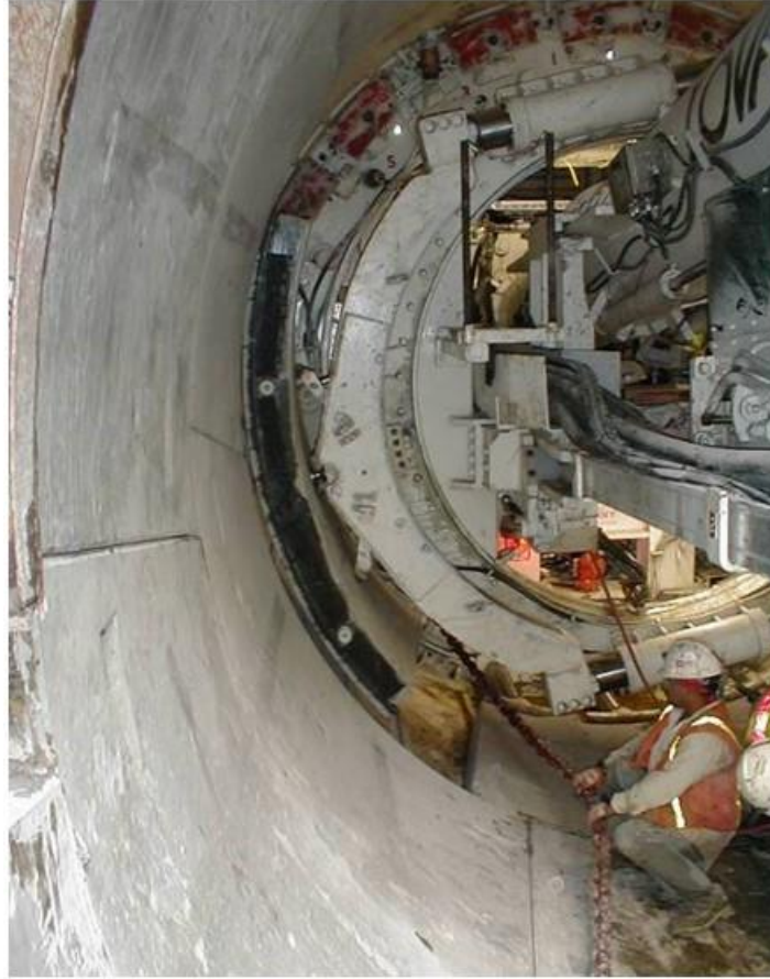
Figure 4. Erecting a Pre-Cast Concrete Segment in Tail of Tunnel Boring Machine
