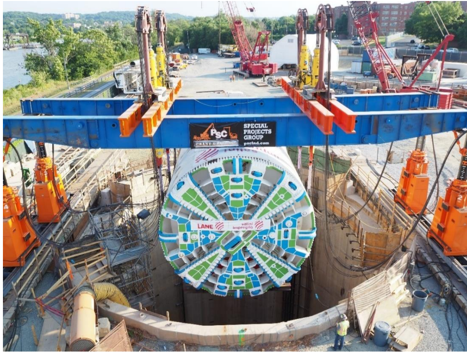
Figure 10. Example of a Large-diameter TBM Being Lowered into a Main Work Shaft
