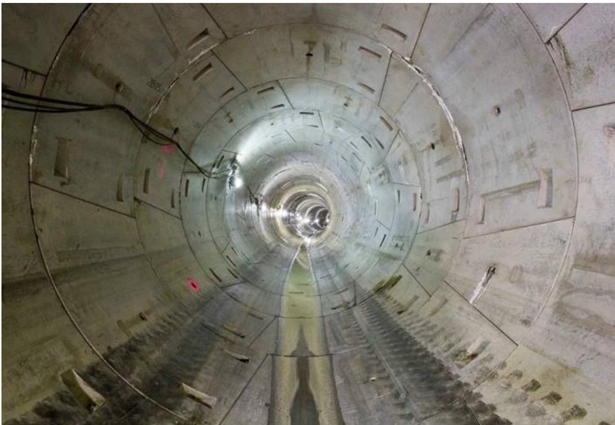
Figure 4. Example Pre-cast Concrete Segmental Lining
