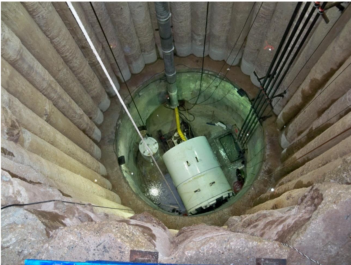
Figure 5. Example of Secant Pile Shaft with TBM
