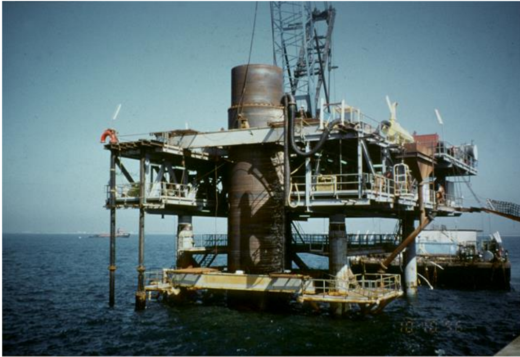
Figure 6. Example of a Vertical Conveyance Shaft Being Lowered Toward a Tunnel at Sea
