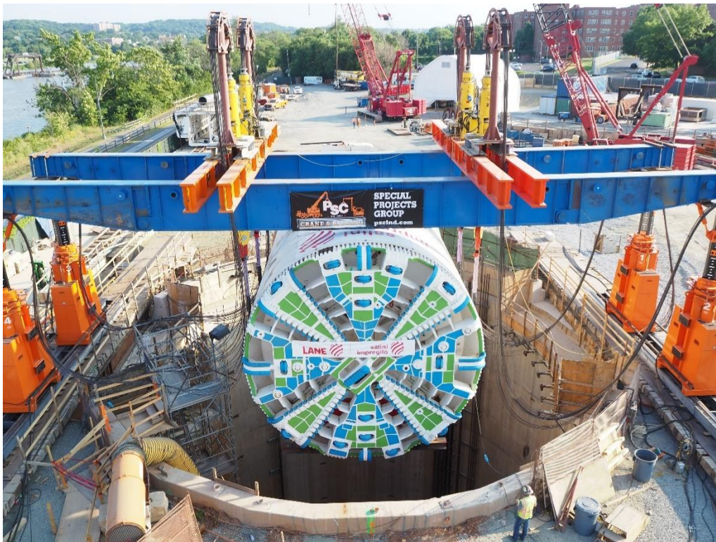
Figure 8. Example of a Large-diameter TBM Cutterhead and Shield Being Lowered into a Main Work Shaft
