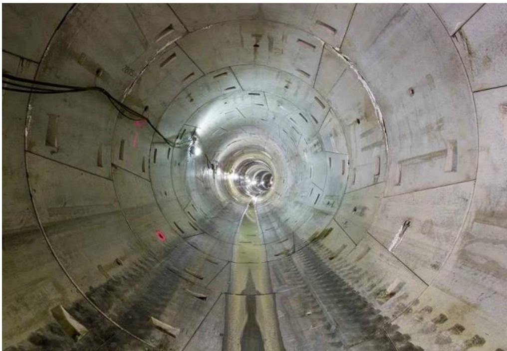
Figure 3. Example Pre-Cast Concrete Segmental Lining
